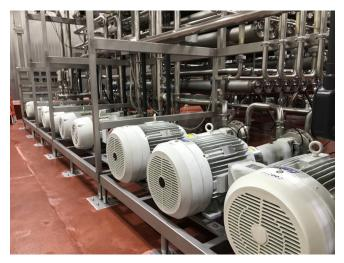
Large centrifugal pumps at the base of this membrane skid push liquid whey through the various membrane banks above. Once a waste product, whey now has numerous commercial uses.
