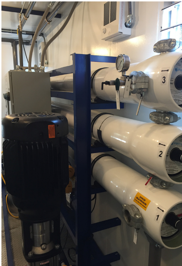
A reverse osmosis step further polishes a portion of the effluent to enable the water's reuse in cooling towers. Michael Mecredy
