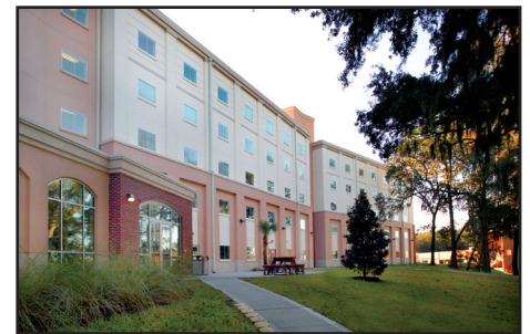
Enhancement JU’s addition includes a 500-bed facility with student suites.
