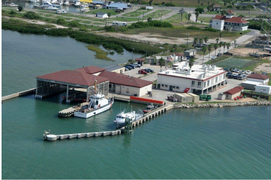
Figure 1-2: Existing USCG STA SPI (photo taken prior to fire, facing NE)
