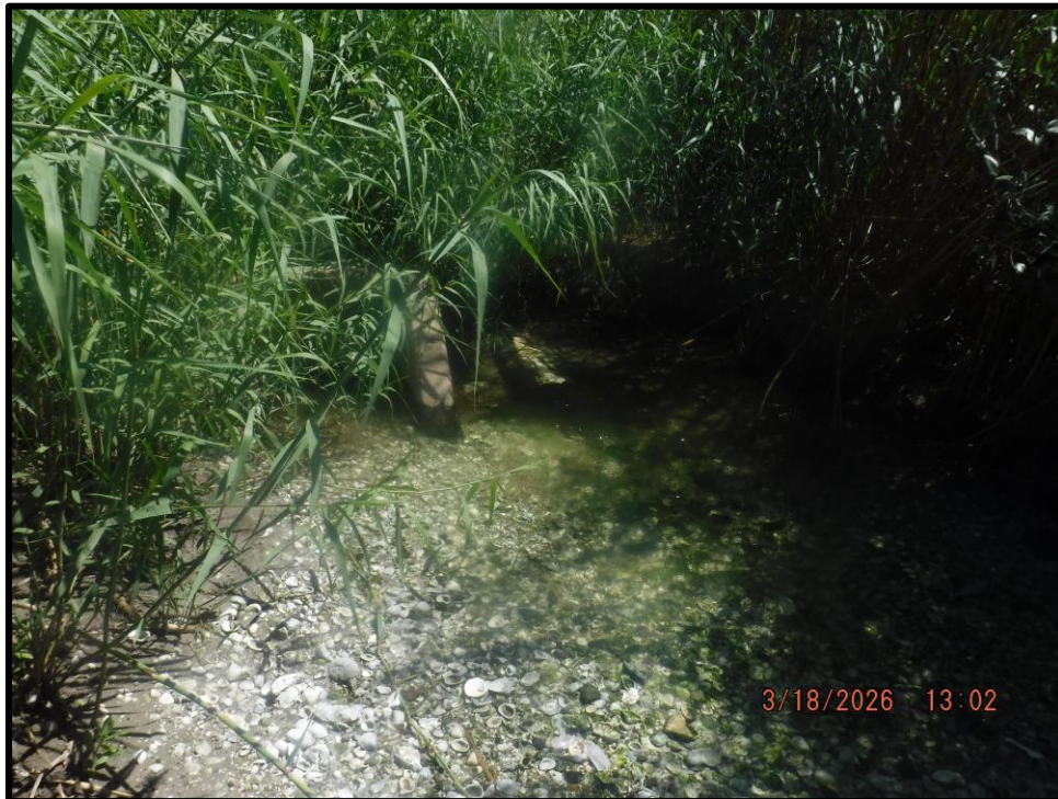
Photo 14: Photo of treated water outfall located within mangrove stand.
