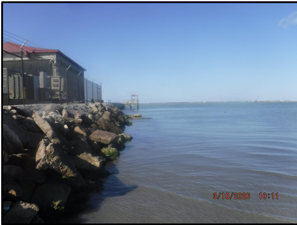
Photo 6: Photo showing rock breakwater wall with subtidal area.
